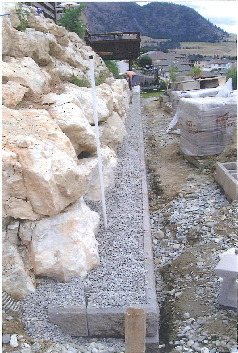
WALLS UNDER CONSTRUCTION LOOKING EAST
