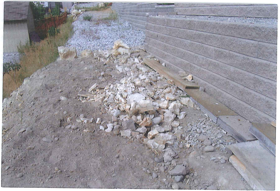
LOOKING WEST ALONG SEWER ROW
